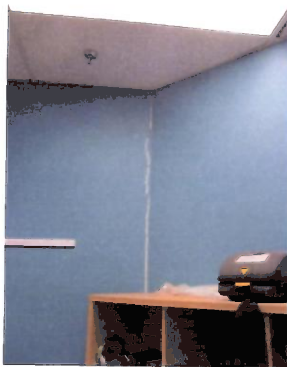
Photo 5: Extensive interior cracking, largely concealed by wall finishes
