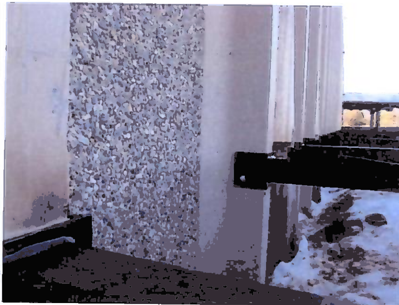
Photo 20: Permanent load introduced into precast, pre-stressed exterior wall panels
