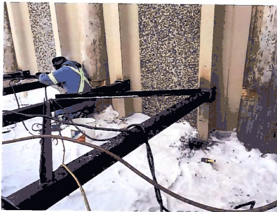
Photo 15: Custom-fabricated structural steel struts installed to brace precast, pre-stressed exterior wall panels
