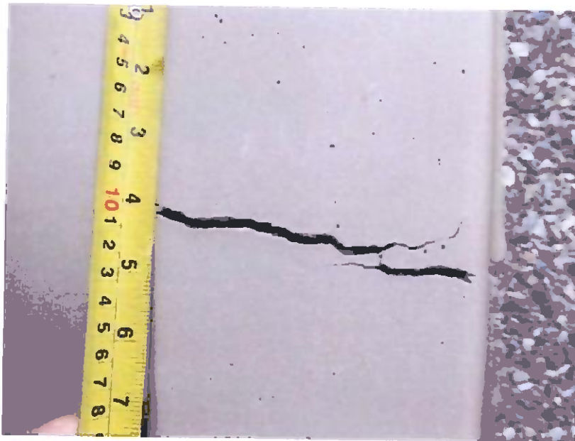
Photo 9: Extensive displacement and cracking of precast, pre-stressed exterior wall panels
