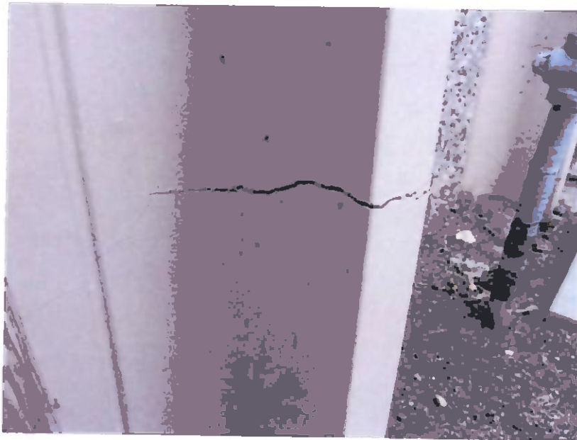
Photo 9: Extensive displacement and cracking of precast, pre-stressed exterior wall panels
