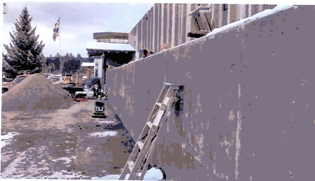
Photo 14: Existing retaining wall removed and new structural buttress constructed (fall, 2015)
