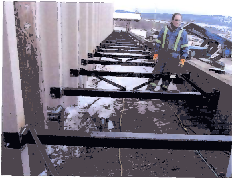
Photo 17: Custom-fabricated structural steel struts installed to brace precast, pre-stressed exterior wall panels
