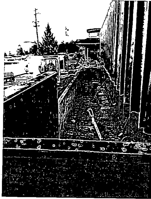
Photo 11: Existing retaining wall removed and new structural buttress constructed (fall, 2015)
