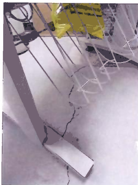
Photo 3: Extensive cracking in cast-in-place slab-on-grade, largely concealed by floor coverings
