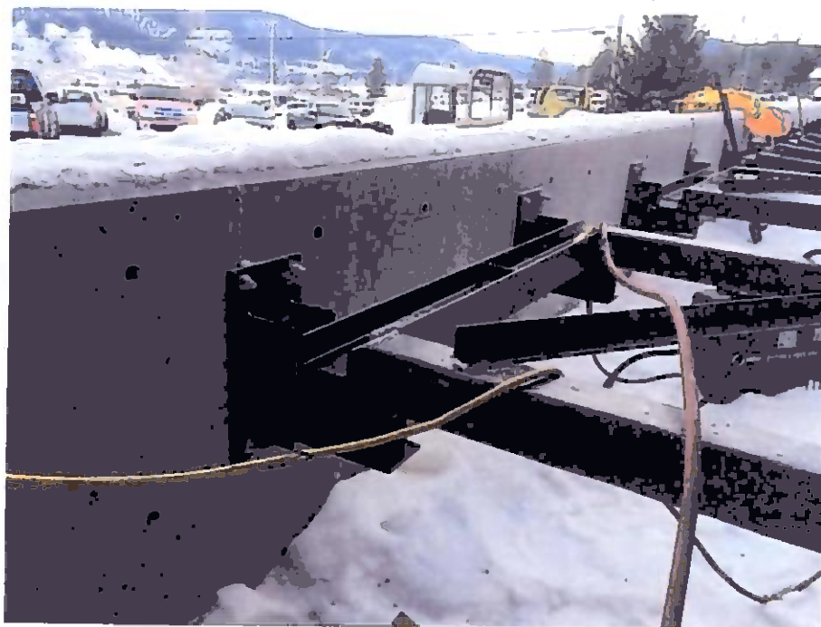
Photo 16: Custom-fabricated structural steel struts installed to brace precast, pre-stressed exterior wall panels
