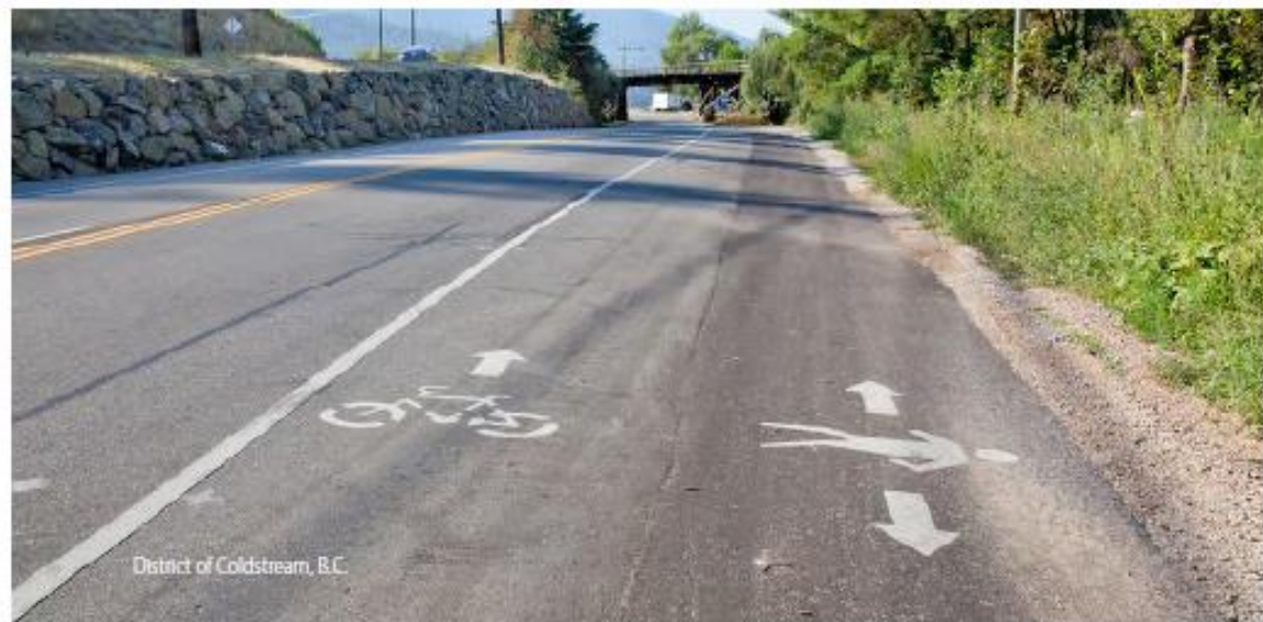
Figure 6. Example of dedicated shoulder for active transportation. BC Active Transportation Design Guide 2019.
