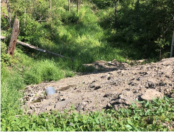
IMAGE 7 – VIEW LOOKING NORTH DOWN THE RUTLEY CREEK GULLY FROM THE EMBANKMENT FILL CONSTRUCTED ACROSS THE GULLY FOR THE TRAILER PARK. RECENT FILL ON THE SURFACE MAY HAVE BEEN PLACE HERE AS A RESULT OF RECENT ROAD WORKS AT SHAW AND DOG CREEK ROADS.
