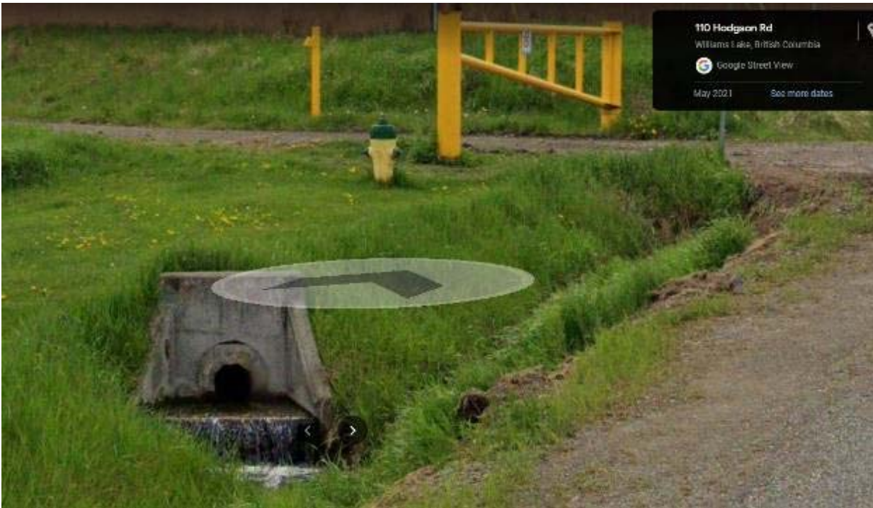
IMAGE 9 – VOLUME OF WATER FLOW CAPTURED FROM THE COMBINED CARSWELL, PERREAULT, AND PRIMA CREEK BASINS BEING DISCHARGED INTO THE HODGSON ROAD DITCH JUST NORTH OF THE RESERVOIR ACCESS ROAD. THIS DRAINAGE SYSTEM IS UNDERSTOOD TO HAVE BEEN INSTALLED BEHIND A RETAINING WALL CONSTRUCTED FOR THE TERRA RIDGE DEVELOPMENT IN THE EARLY TO MIDDLE OF THE 1990s. IT IS UNDERSTOOD THAT WORK WAS DONE ON THE WALL AND DRAINAGE SYSTEM IN AROUND 2019.
