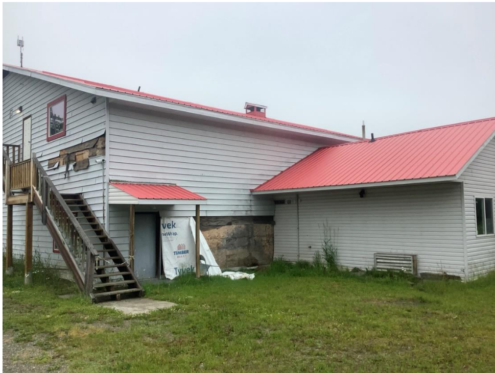
Figure 7: Forest Grove Fire Department Hall 1. Damaged siding exposing flammable underlay, tall vegetation adjacent to building and untreated wooden staircase on exterior identified by Forsite staff during CWRP Wildfire Threat Assessment fieldwork.
